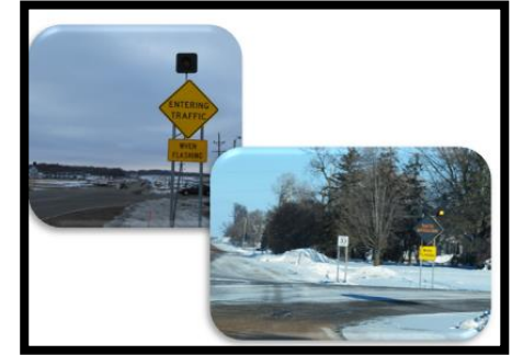
Dynamic Warning Signs
